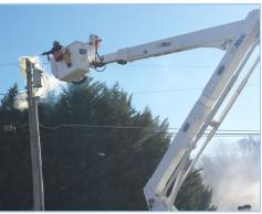
The photo shows an AUB lineman using a hand-held fire extinguisher to put out the flames.
